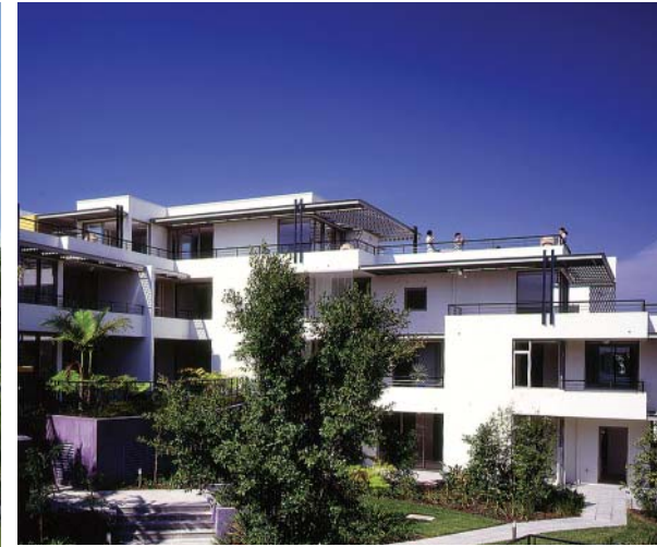
Figure 61: Stepped building forms respond to topography and views.
